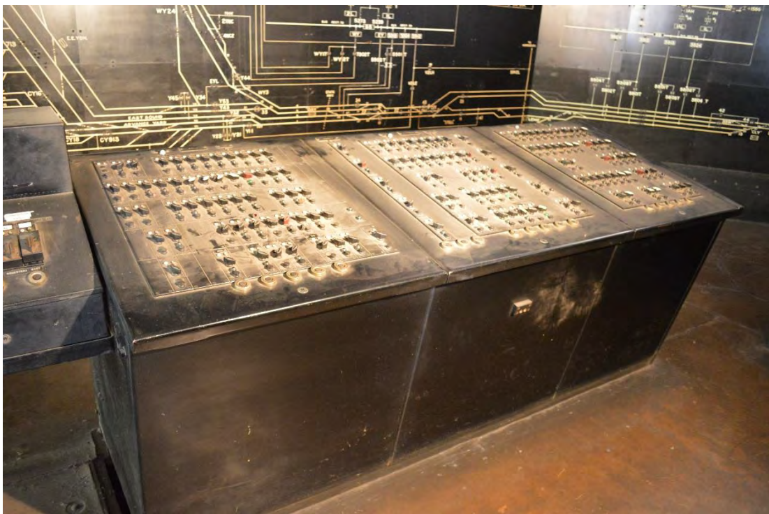
Photograph 10: Westinghouse three-panel console.
