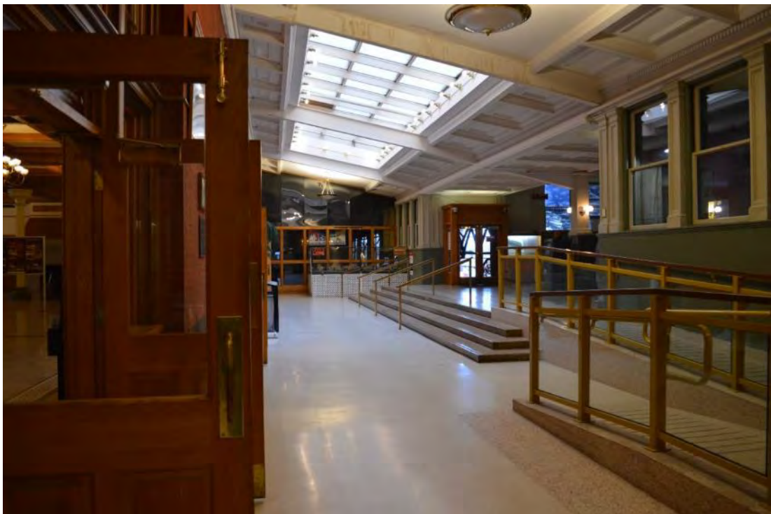
Photograph 33: View of hall between waiting area and concourse, showing skylights, looking north.
