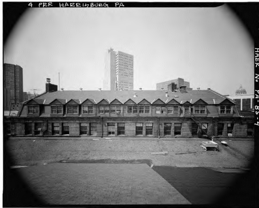
Image 39: Partial view. Looking from shed roof, of rear (east) elevation, showing second and third stories of original section. (HAER 1985)
