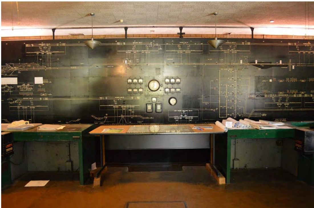
Photograph 12: Two Kellogg Switchboard & Supply Co. signal control units.
