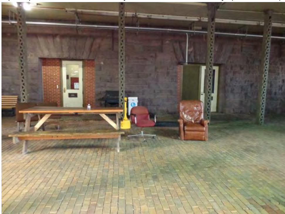
Image 38: Similar view, showing masonry base and lattice columns at the basement (track) level, 2017.
