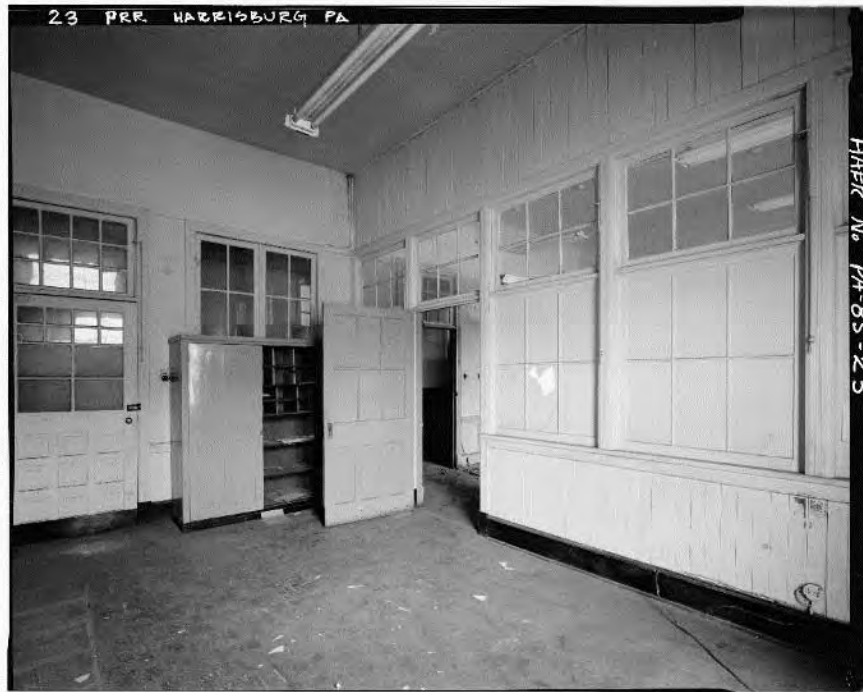
Figure 13: 1981 photograph of a typical second floor office (HAER PA-85-23).
