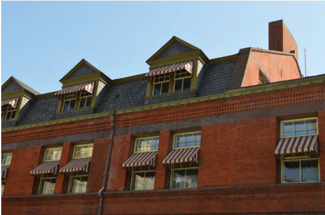
Photograph 9: Detail of passenger station facade, showing upper story windows and dormers, looking east. Note the terra cotta dentil molding details.
