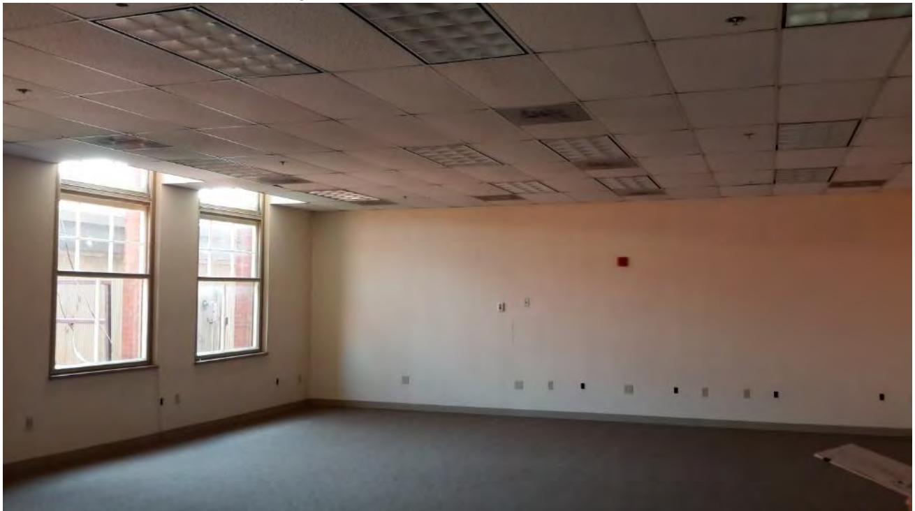
Image 46: View of a third-floor office space, 2016.
