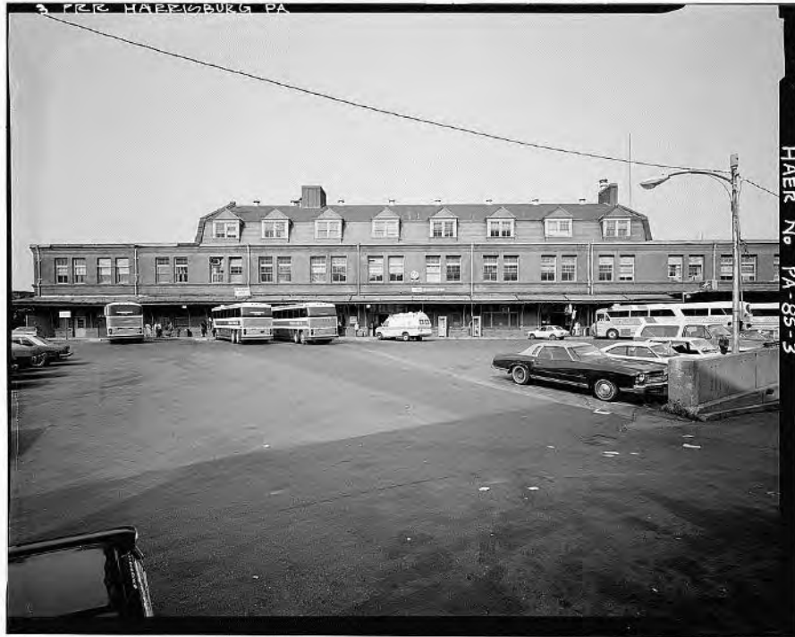
Image 5: View of front (west) elevation. (HAER 1985)
