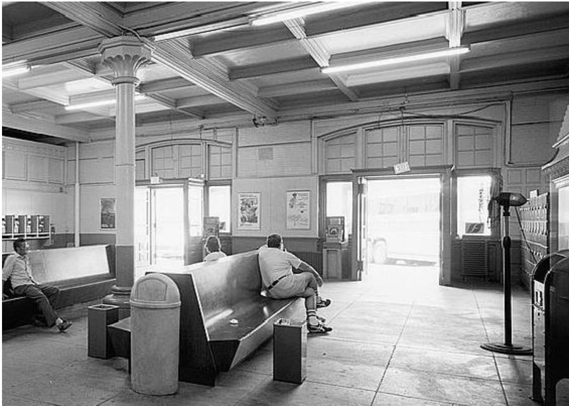
Figure 9: Detail of a 1981 photograph showing interior entrance vestibules (HAER PA-85-9).
