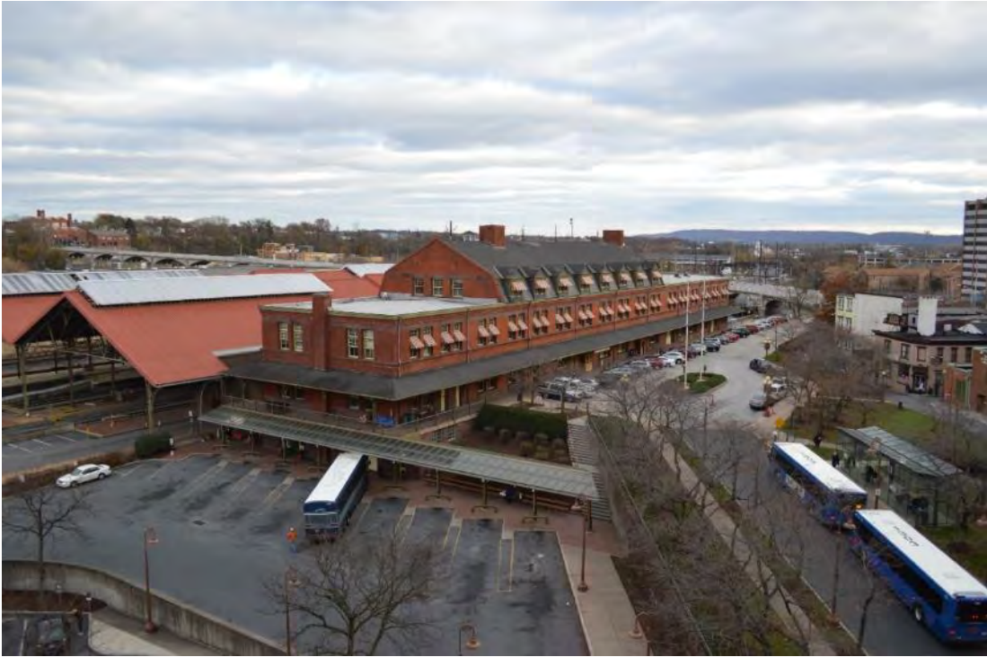
Photograph 1: View of the passenger station and train sheds, looking southeast.
