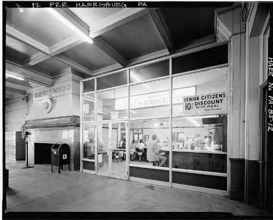
Image 19: Detail view of north wall, main waiting room, first floor. Note fireplace and luncheonette entrance. (HAER 1985)
