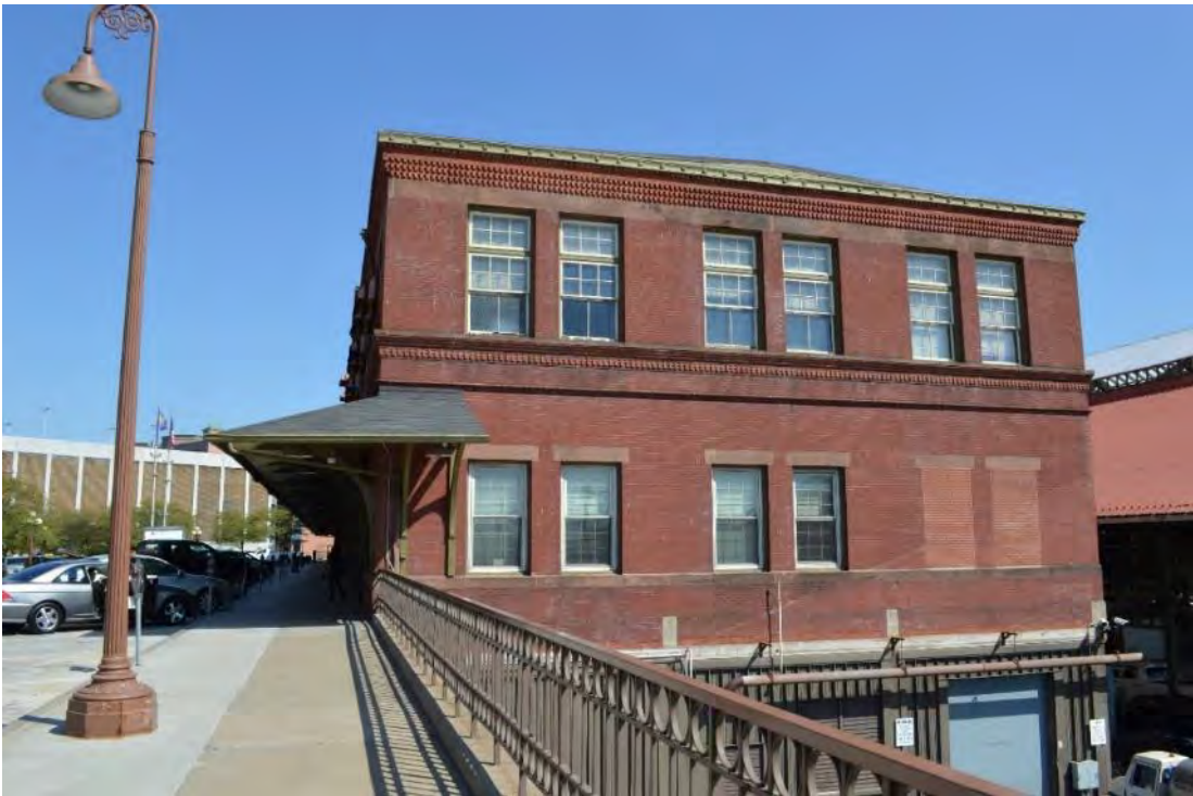
Photograph 6: View of passenger station's south elevation, looking north.
