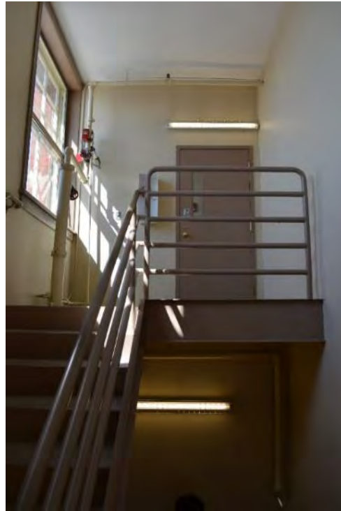
Photograph 50: View of stairway between second and third floor, looking north.
