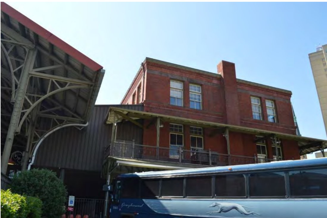
Photograph 12: Detail view of the north facade of the passenger station, showing the train shed trusses and the station canopy, looking south.
