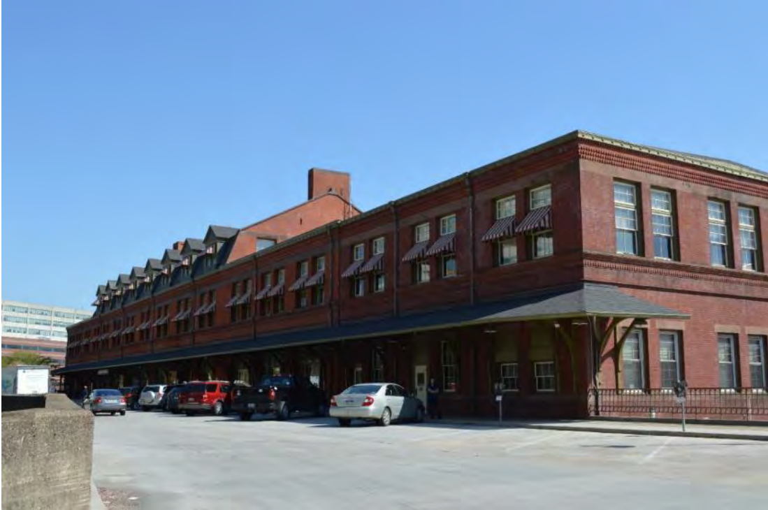
Photograph 5: View of passenger station with 1937 south addition in the foreground, looking northeast.
