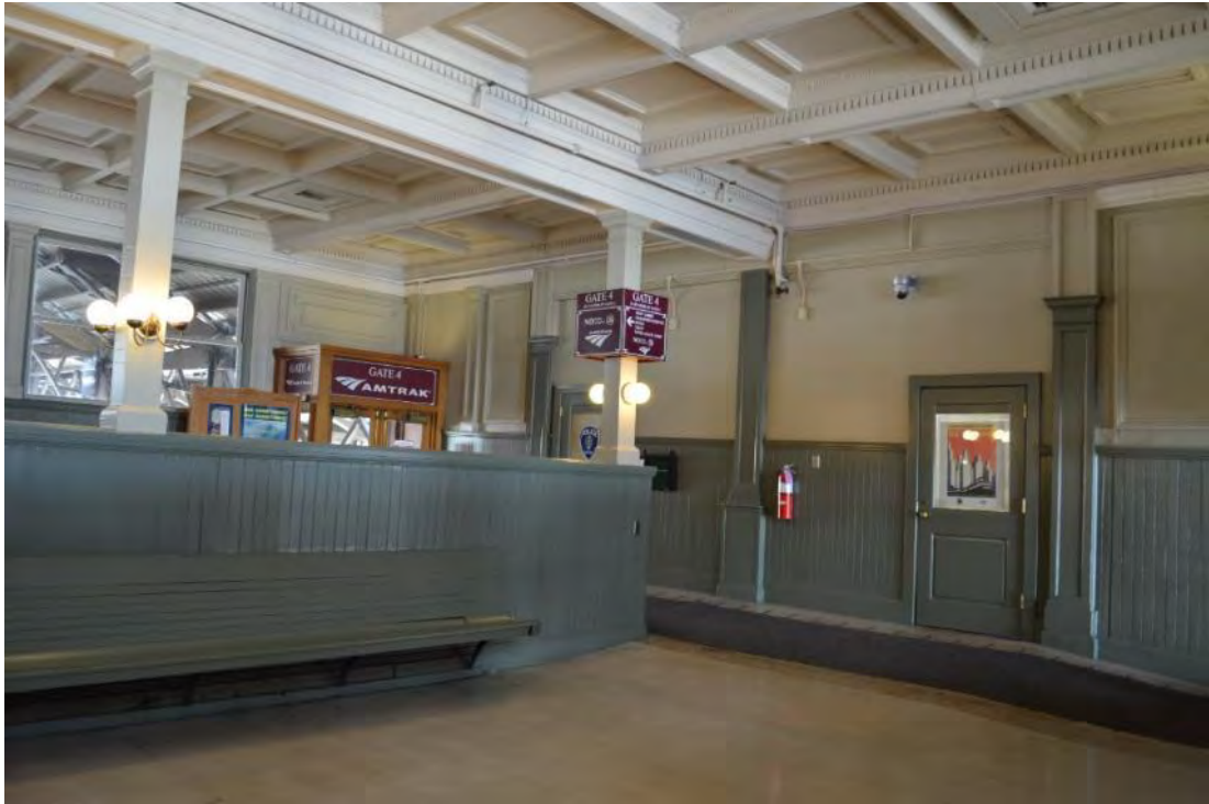
Photograph 36: View of concourse partition wall, looking northwest.
