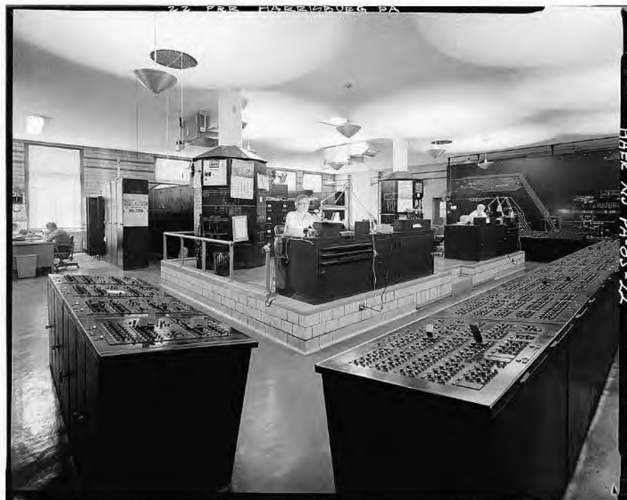
Image 30: Overall view of power directors room, second floor. (HAER 1985)
