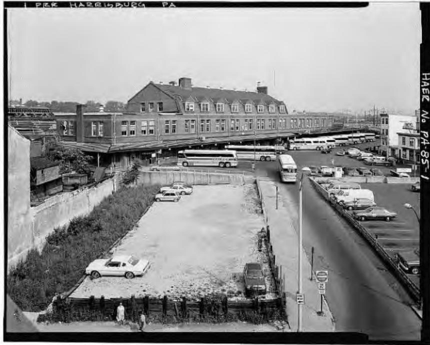
Image 1: View of northwest approach, showing existing parking lot in front of passenger station and bus staging area. (HAER 1985)
