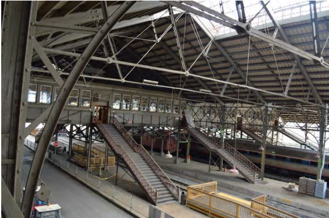
Photograph 15: Exterior view of passenger bridge, looking northeast.
