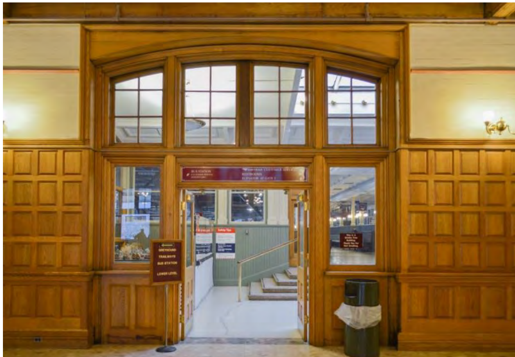
Image 48: Detail view from west of the east wall of the main lobby, 2017.
