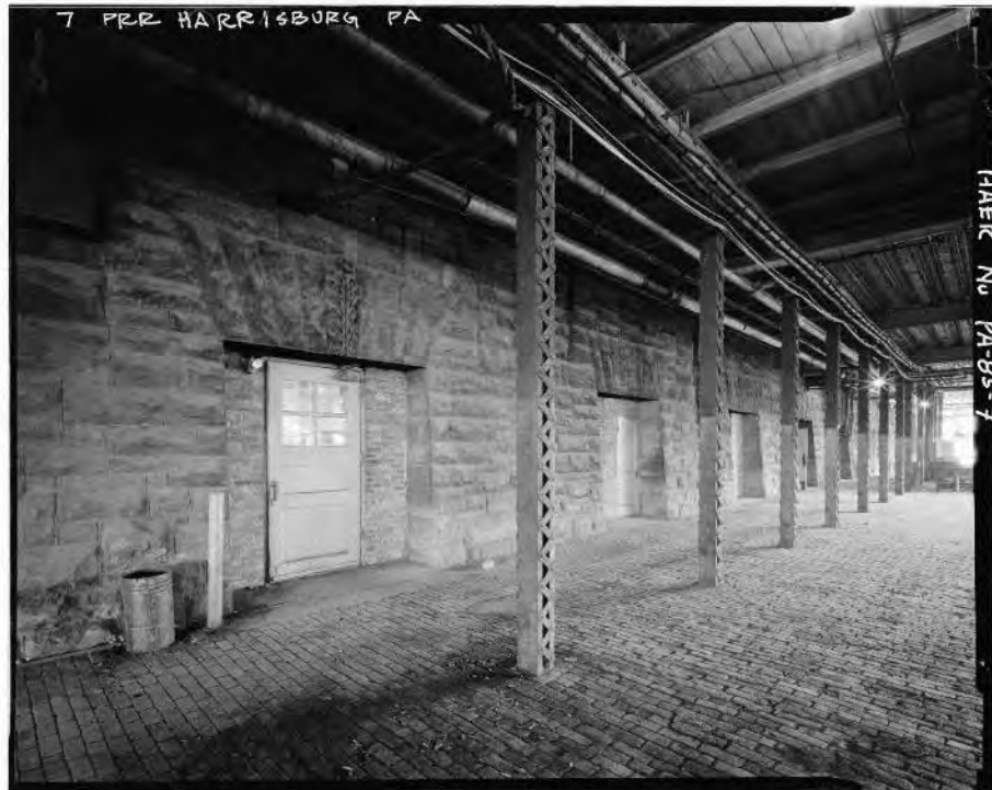
Image 37: Partial view of rear (west) façade, showing masonry base and lattice columns at basement (track) level. Note acanthus keystone detail over doorway. (HAER 1985)
