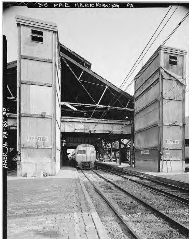
Figure 15: 1981 photograph showing the passenger bridge and elevators (HAER PA-85-30).
