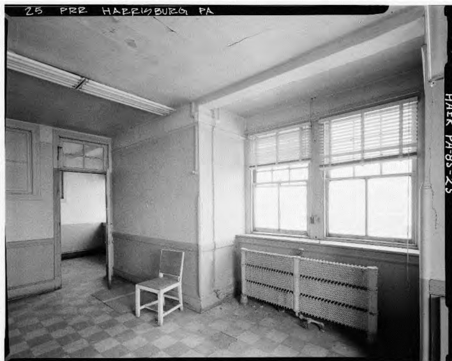
Image 42: View of a typical office, third floor. Note dormer offset of rear façade. (HAER 1985)
