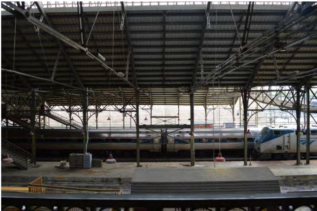
Photograph 16: View of former location of baggage bridge, demolished 2018, looking east.
