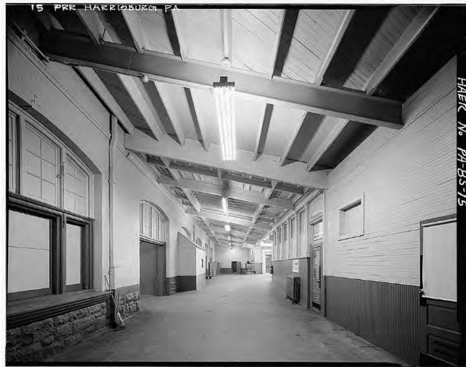
Image 25: View, from south end, of new lobby, first floor. Note exterior walls of the original section at left. (HAER 1985)
