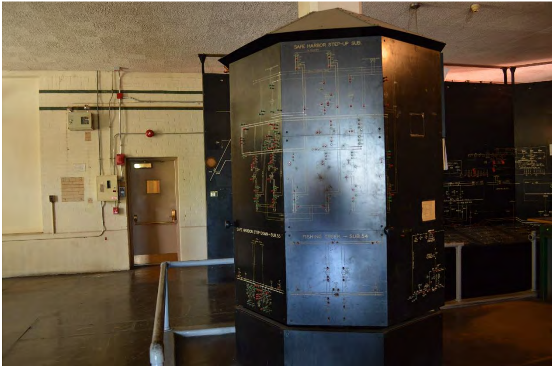
Photograph 6: General Electric Octagonal Display (1 of 2).
