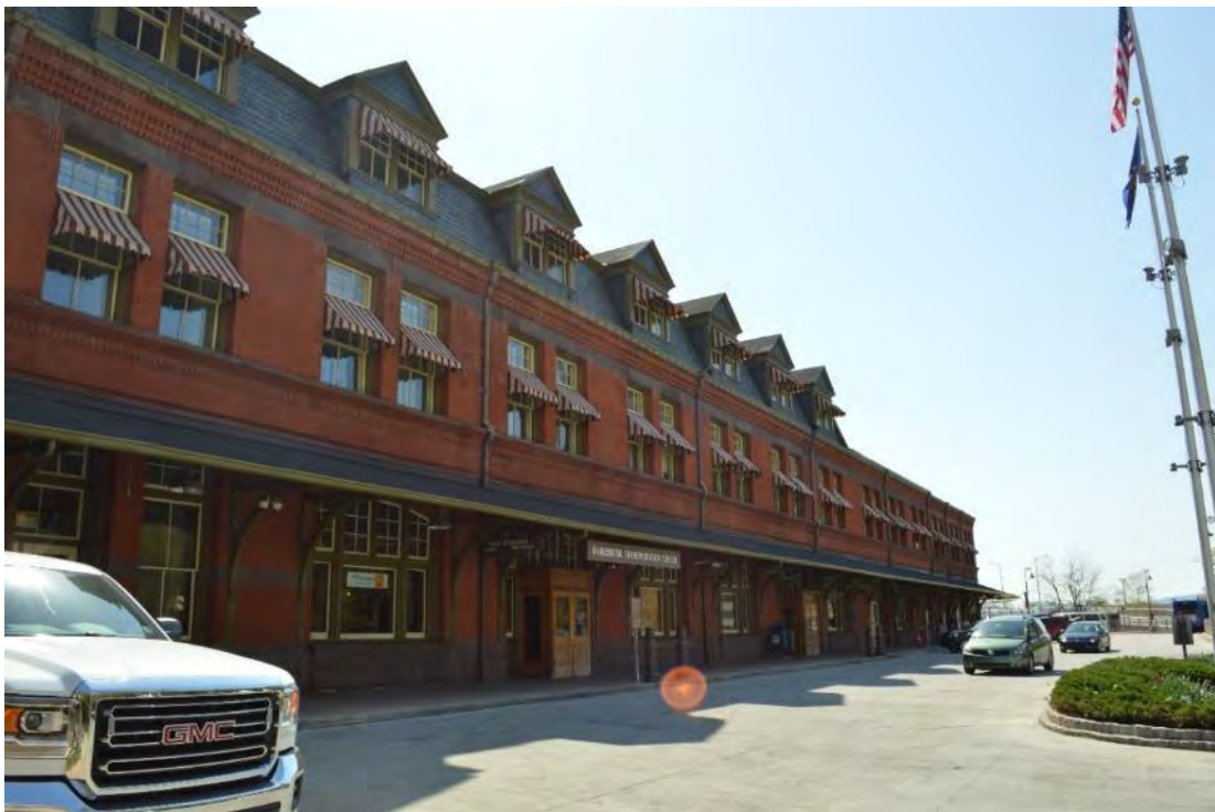
Photograph 8: View of passenger station, looking southeast.
