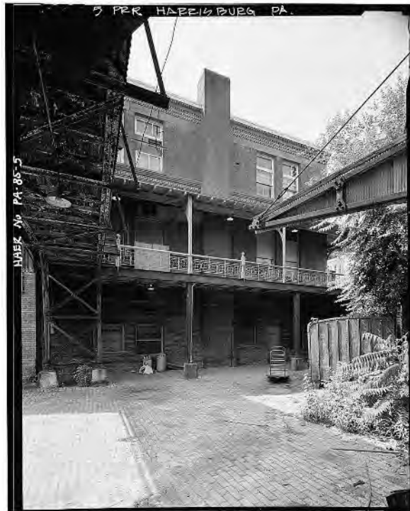
Image 7: View of north elevation, showing bridging connecting the station building with the Hoffman House at upper left. Note balcony which meets the front plaza level at right. (HAER 1985)
