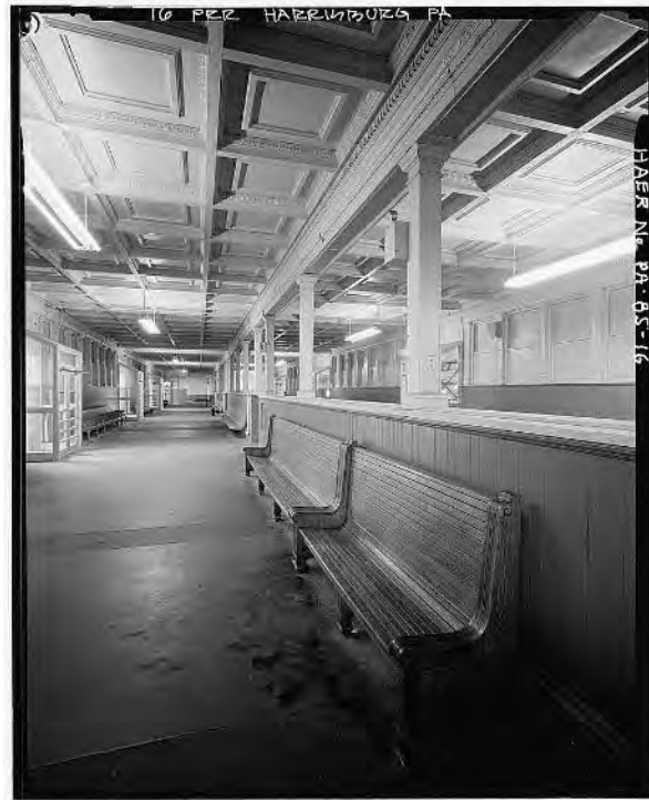
Image 27: View, from new lobby, of concourse, first floor. Note exits to platforms. (HAER 1985)
