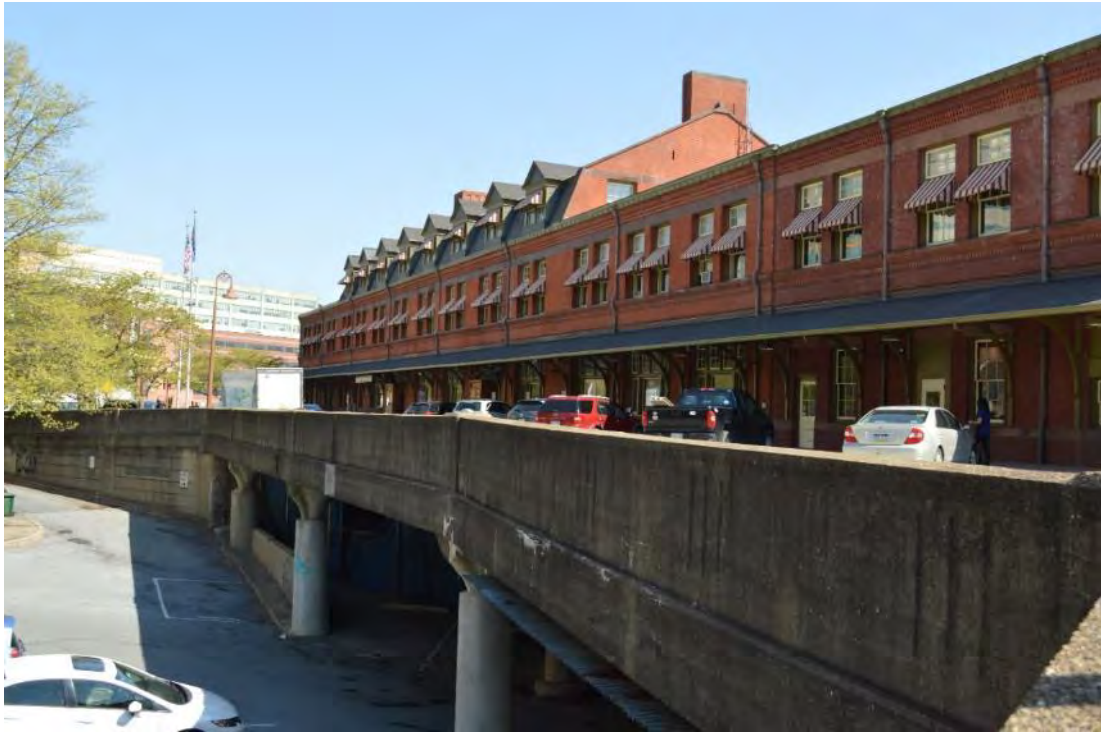
Photograph 7: View of passenger station and viaduct, looking northeast.
