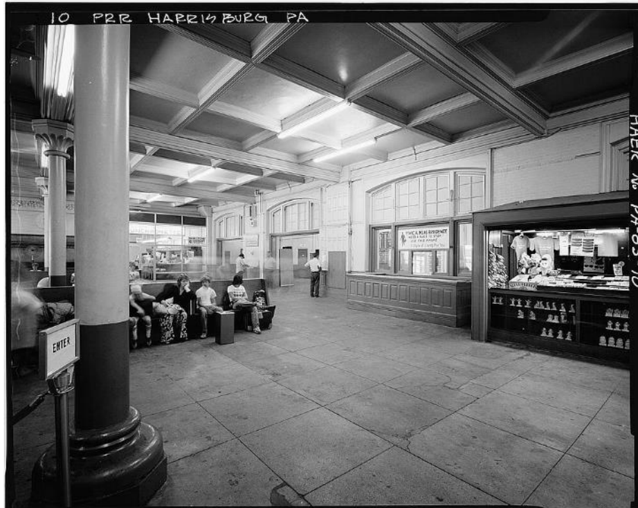
Figure 10: 1981 photograph of waiting room (HAER PA-85-10).
