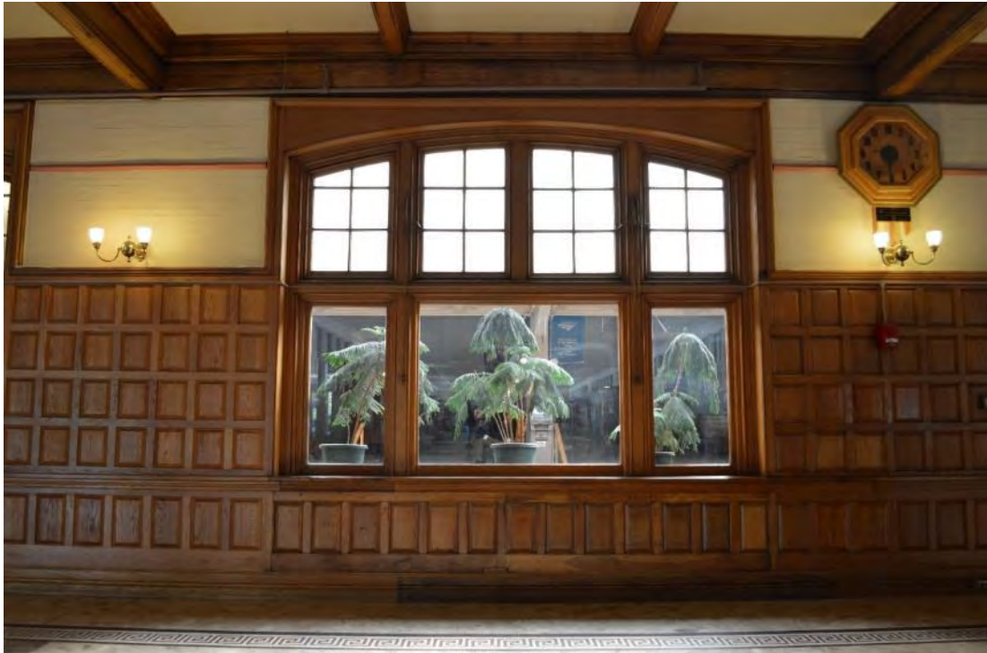
Photograph 22: Detail of main waiting room windows between main waiting room and concourse, looking east.
