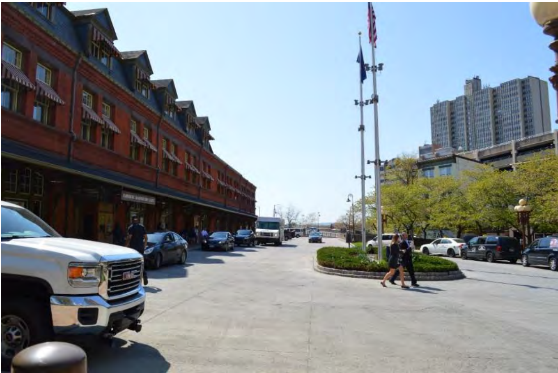
Photograph 4: View of plaza at front of passenger station, looking south.
