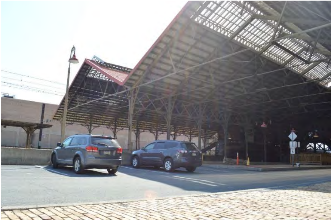
Photograph 13: Detail view of train sheds, looking east.
