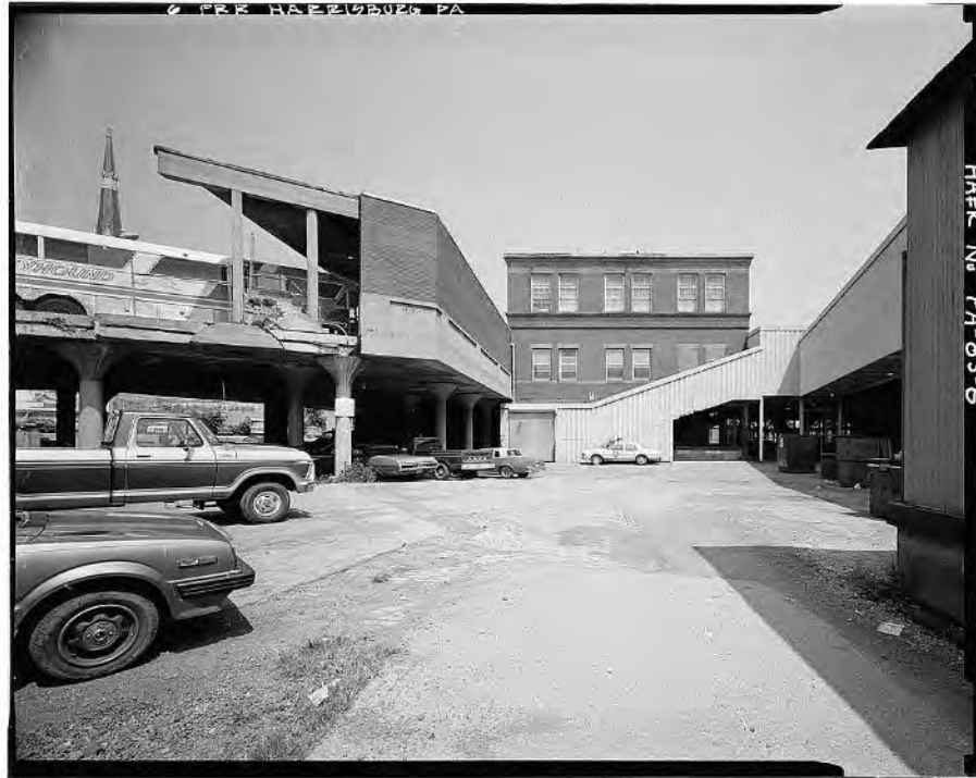
Image 9: View of south elevation, showing viaduct connecting to parking lot and bus staging area at plaza level over staff parking area at track level. Note corrugated metal housing of mail conveyor across building façade. (HAER 1985)
