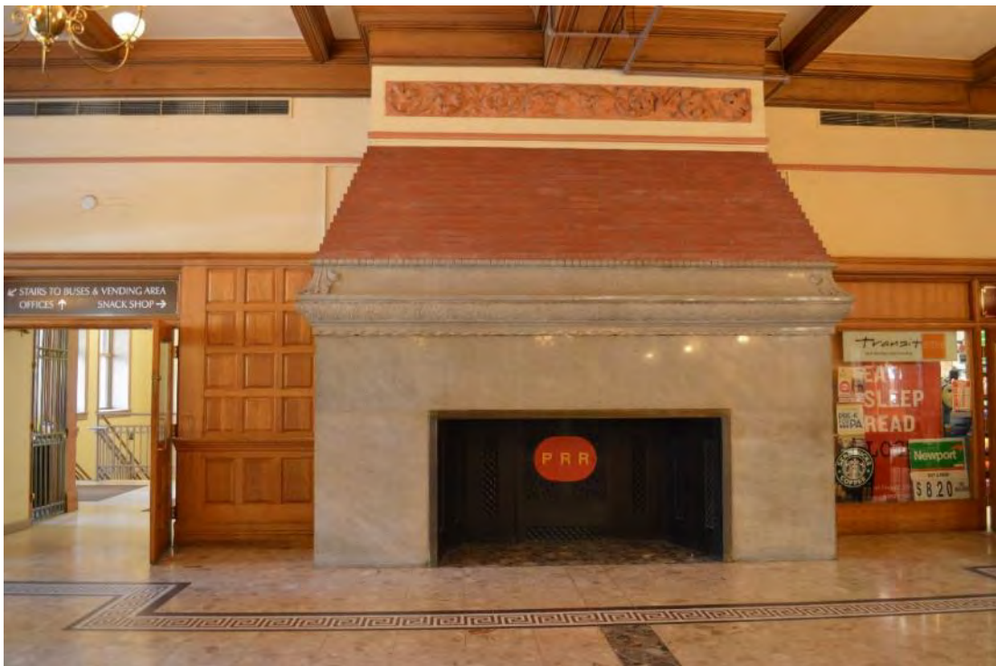
Photograph 27: Fireplace detail, looking north.
