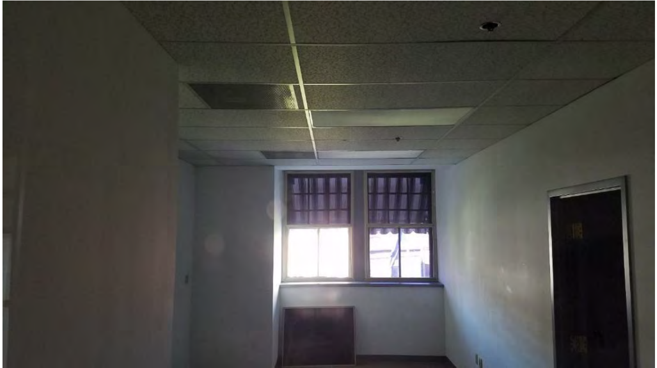
Image 43: View from an office of a dormer window, third floor, 2017.
