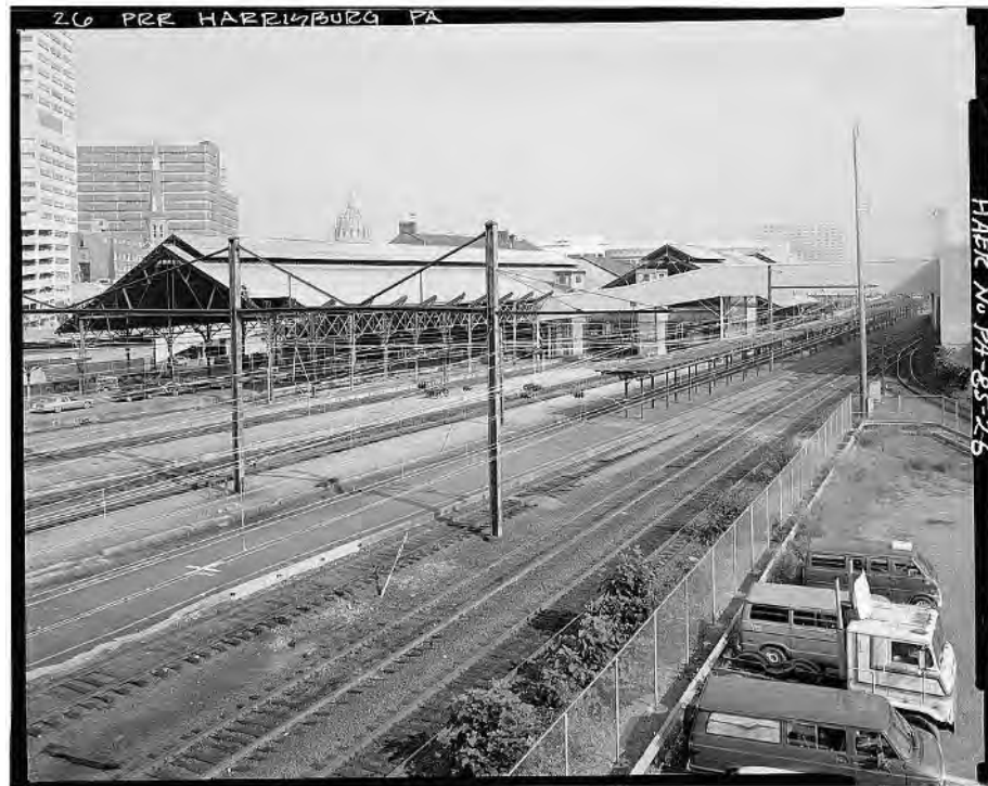
Image 33: Overall view, from south, of Mulberry Street bridge, showing both sheds, mail conveyor connecting post office building to loading dock under west shed (right side), platform canopies and catenary system. Note State Capitol dome visible beyond station building. (HAER 1985)
