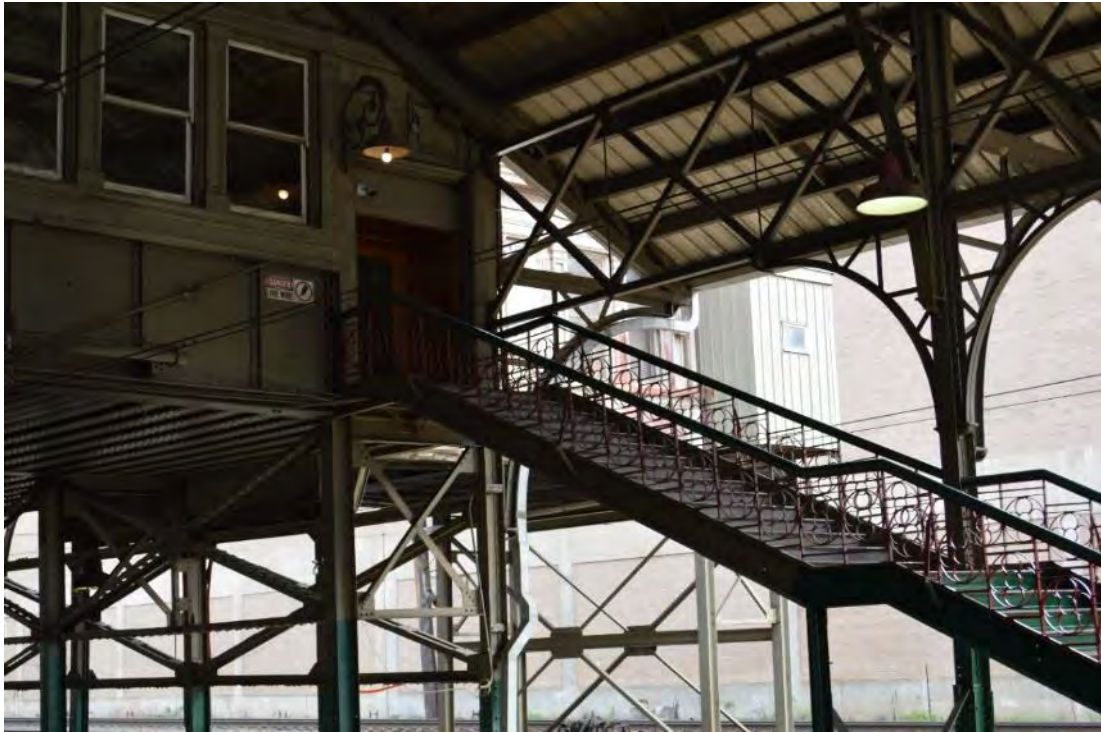
Photograph 17: Detail view of passenger bridge stair, looking northeast.
