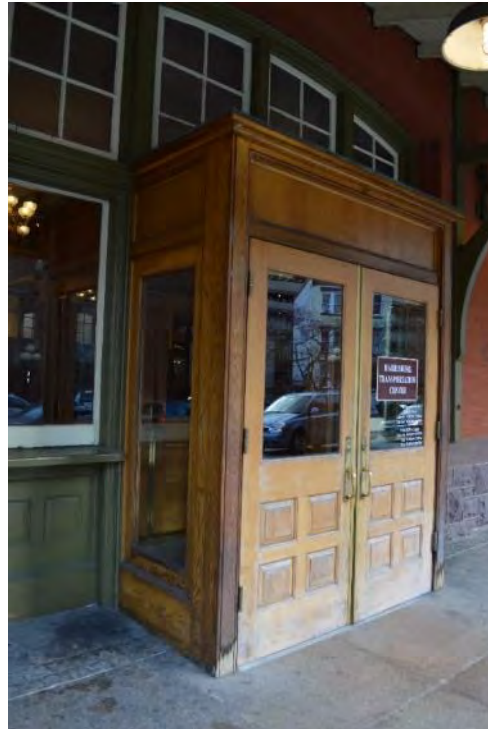
Image 49: Detail view of façade (west), showing vestibule, 2017.
