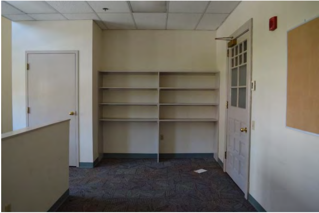
Photograph 46: View of a second-floor office, looking north.
