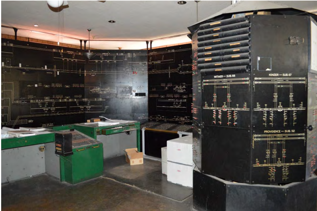
Photograph 7: General Electric Octagonal Display (2 of 2).
